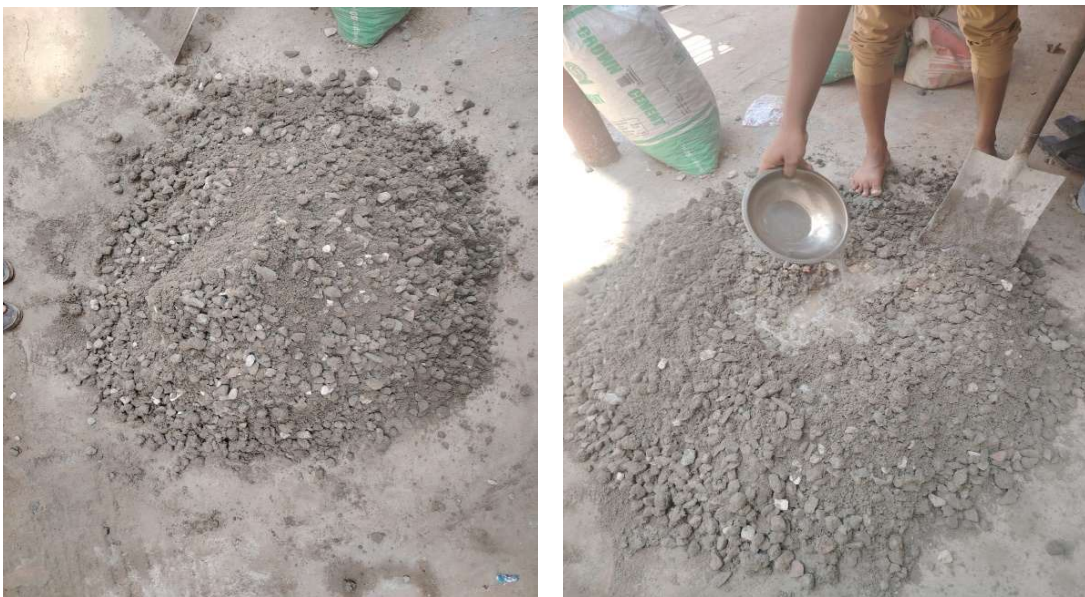
Figure 3.7 Concrete mixing
