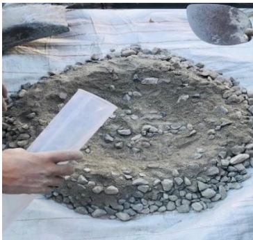
Figure 3.14 Preparation for Concrete Mixing
