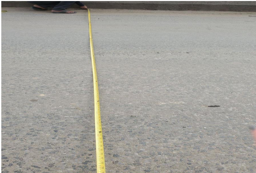
Figure 2.1: Road Width Measurement
