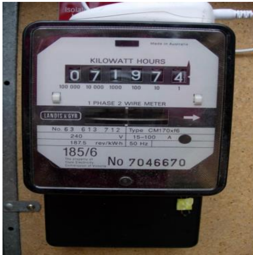
Figure 3.4: Traditional Electricity meter
