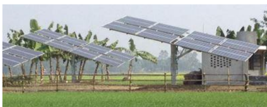
Figure 2: Irrigation system using solar Energy
