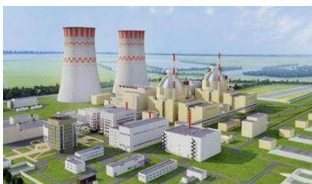
Figure 10: Rooppur proposed nuclear power plant
