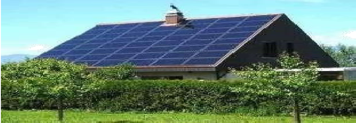
Figure 2.9.a.: Flush Mounting on roof
