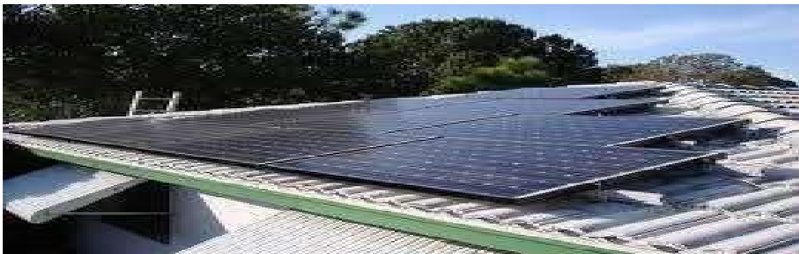
Figure 2.9.c: Fin mounting on roof
