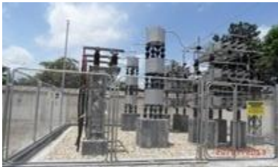
Figure 5.1: Capacitor-bank
