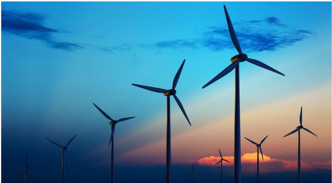
Fig-2.1: wind power plant
