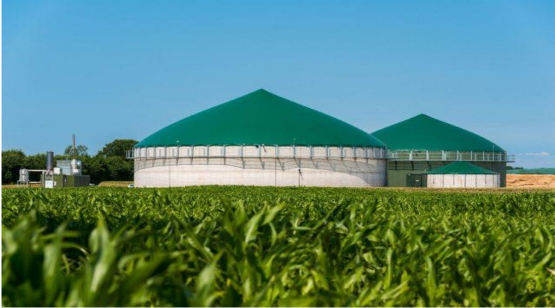
Fig-2.3: Biogas plant
