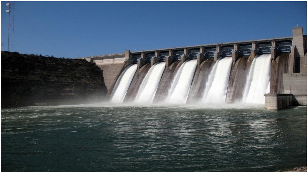
Fig-2.4: Hydro power plant
