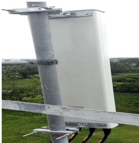
Fig4.22 GSM Antenna
