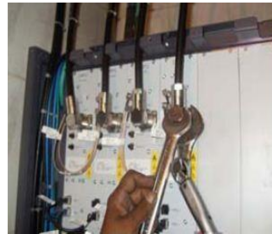
TIGHTEN THE CONNECTOR WITH TORQUE
