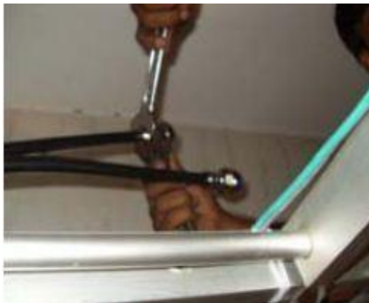
TIGHTEN THE CONNECTOR PROPERLY
