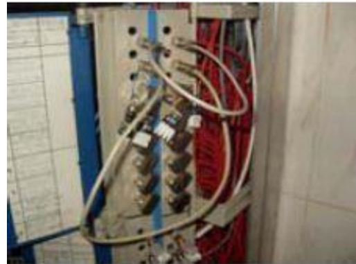
Give a loop for cross checking the E1 path
