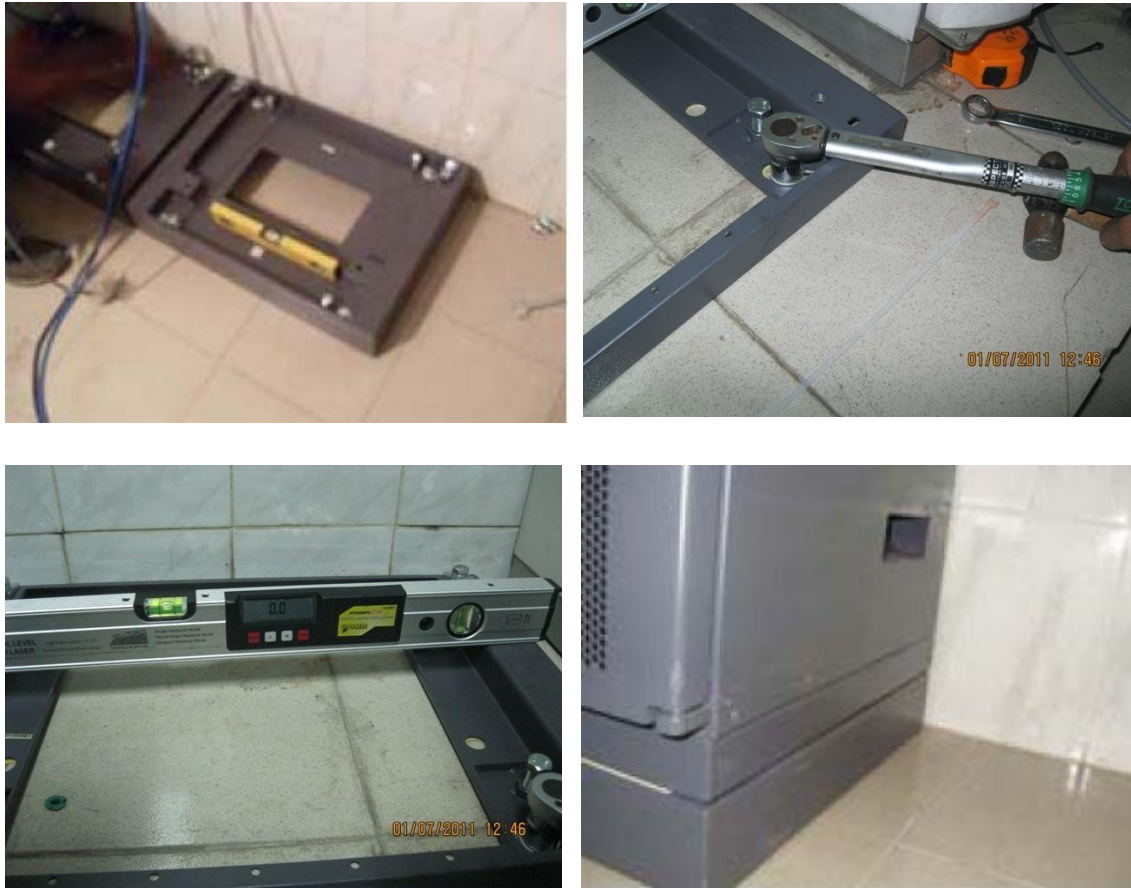
Fig-6.18: Fixing the Huawei BTS and install BTS over base
