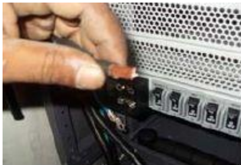
CUT THE ISOLATION OF POWER CABLE
