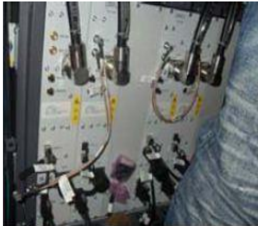
CONNECT THE SUPER FLEX JUMPER AT BTS END
