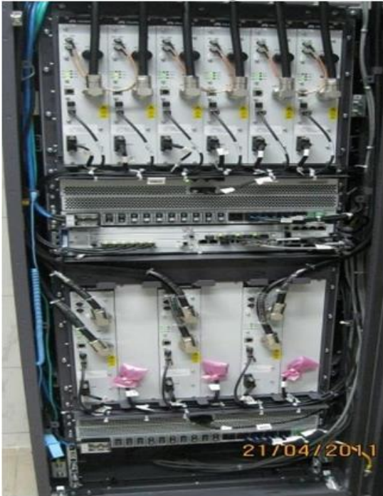
Fig. 6.3 BTS 6900L component
