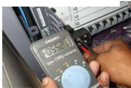
Give a loop for cross checking the E1 path
