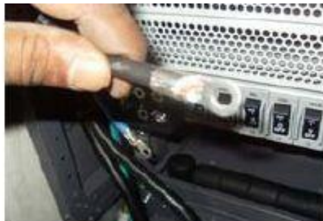
USE PROPER CABLE SHOE
