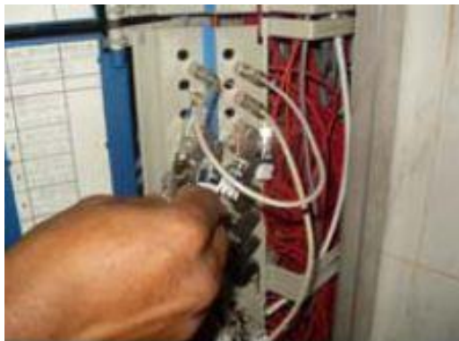
REMOVE THE U-LINK & GIVE A LOOP FOR CROSS CHECKING THE E1 PATH
