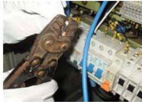
CRIMP THE LUG USED FOR POWER CABLE
