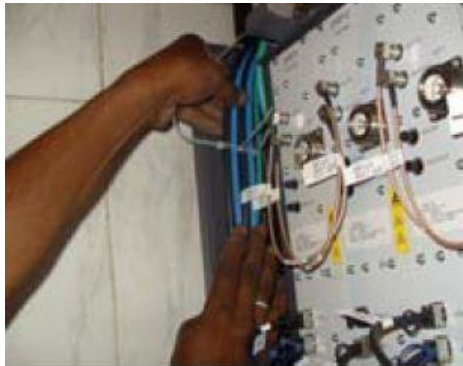
LATCHING THE POWER CABLE AT BTS END
