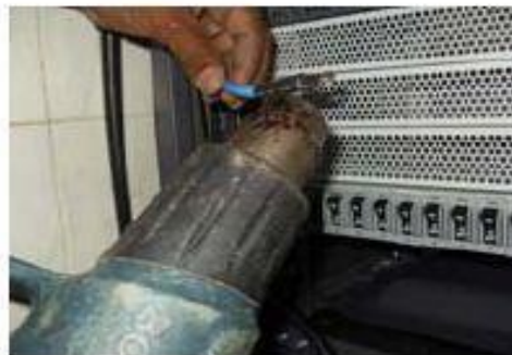
USE HEATSHRINK FOR CABLE SHOE
