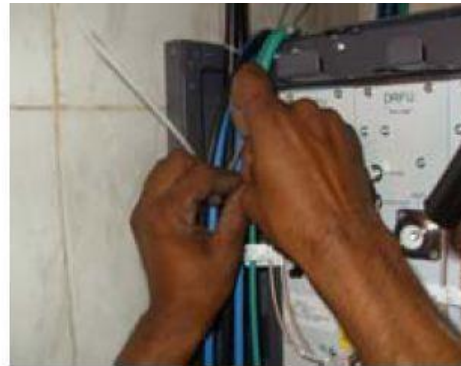
LATCHING THE POWER CABLE AT BTS END
