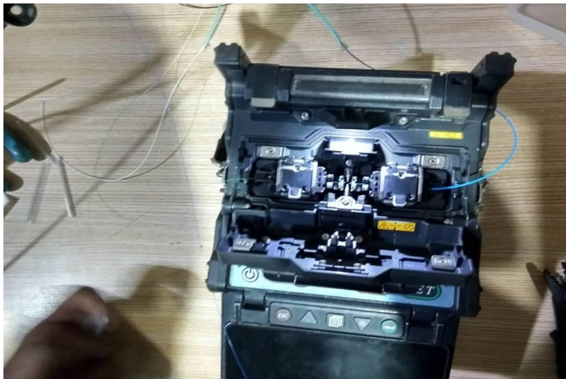
Fig 4.4: Fiber Splicing in Fusion Machine.
