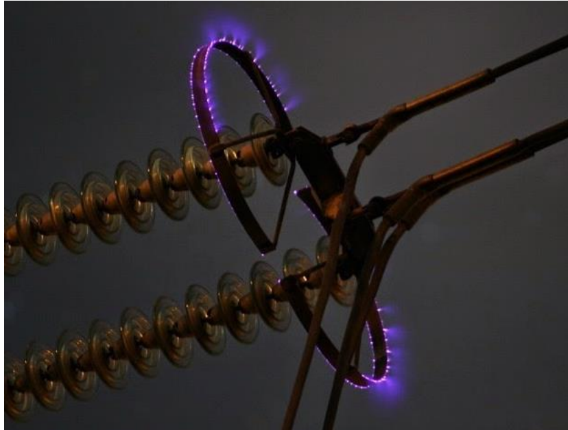
Fig- 4.1: Corona Discharge in Transmission Line
