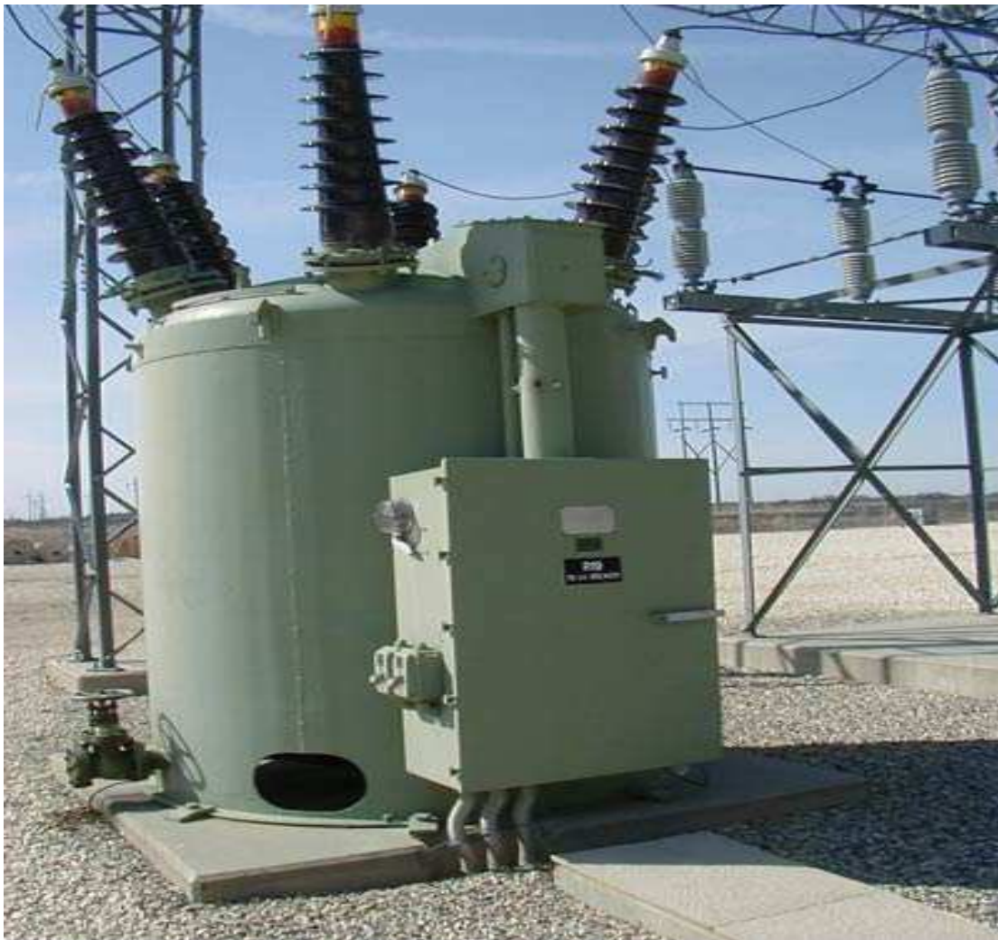
Figure 4.8: The image of SF6 Gas Circuit Breakers.
