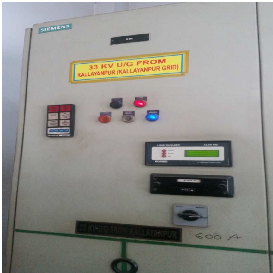
Figure 4.5: 33KV incoming panel-1 (Rampura Grid).
