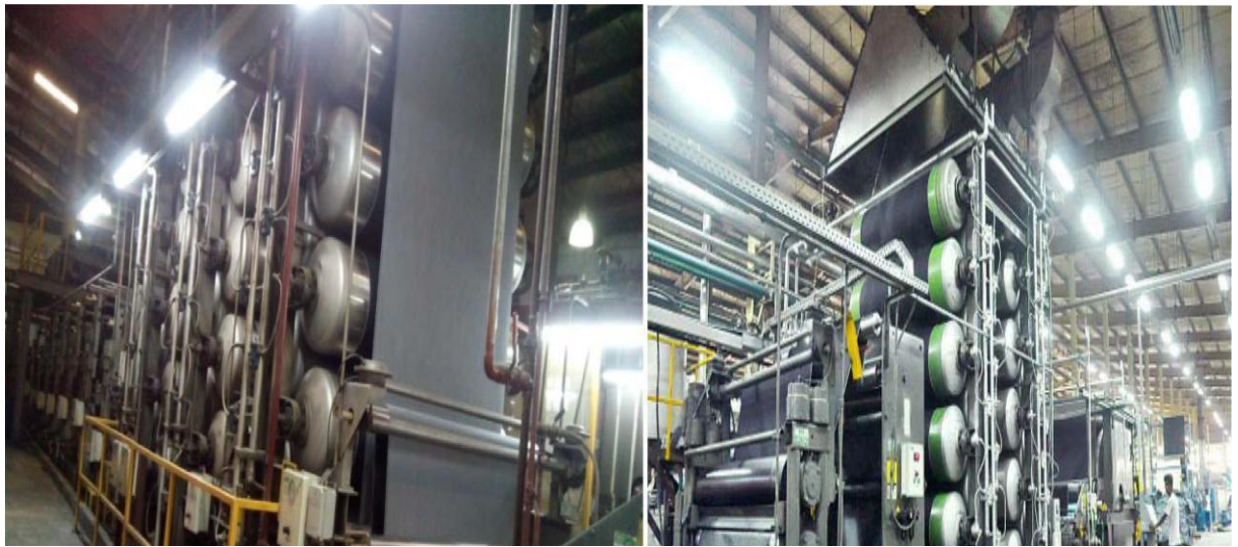
Fig : Finishing section
