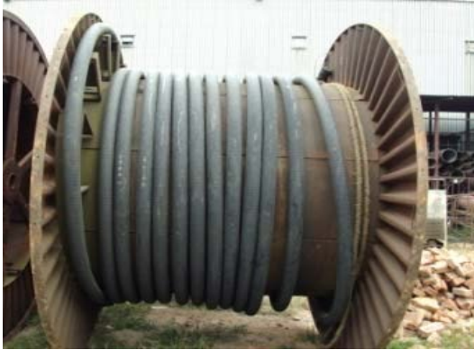
Figure 5.11: XLPE insulated Underground Power Cable used in APSCL
