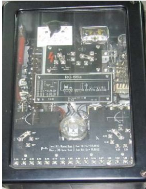
Figure 4.6.4: Under frequency relay.
