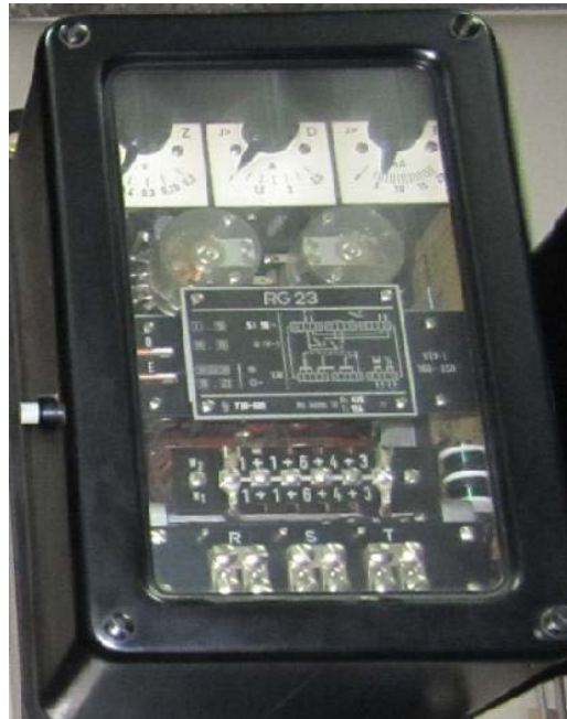
Figure 4.6.8: Generator Differential Relay.
