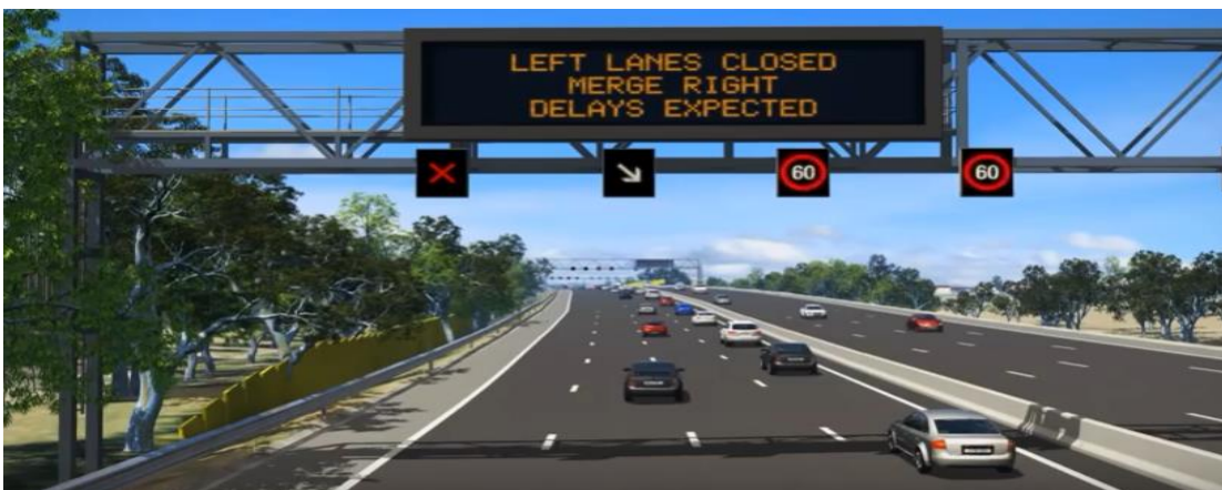
3.8: Ramp Meter System Of Corridor.
