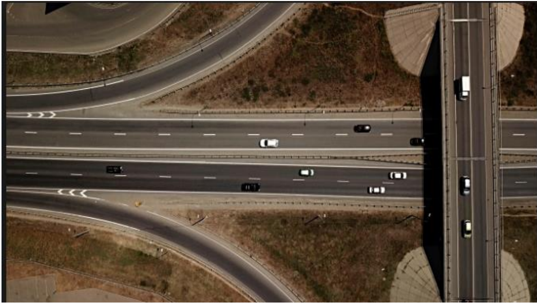
Fig 3.3 : Picture Of I-394 Corridor.
