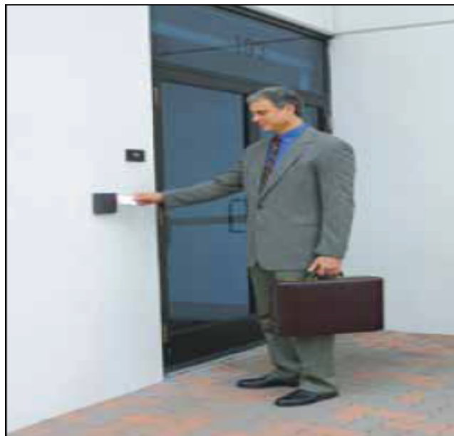
Figure 2.2: A user is trying to open the door by placing an RFID tag near the RFID reader
