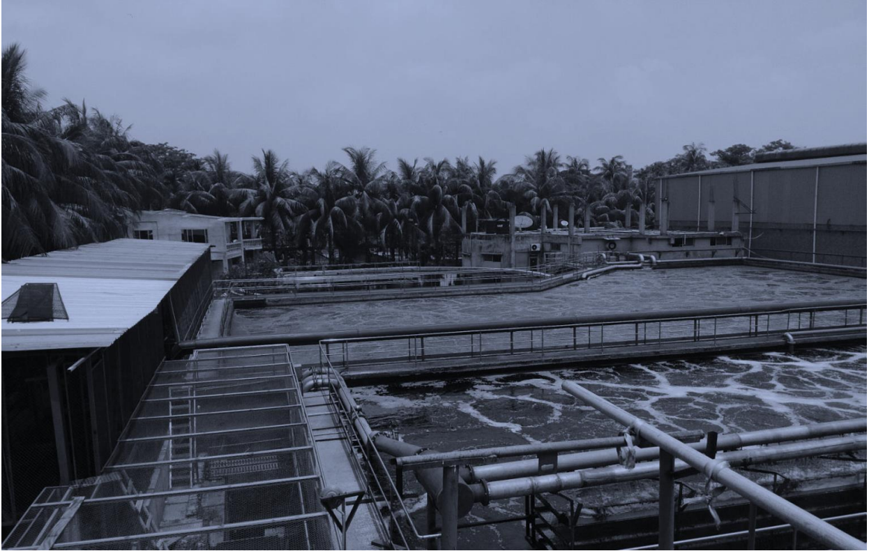
Effluent Treatment Plant
