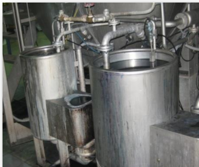
Fig: Addition tank
