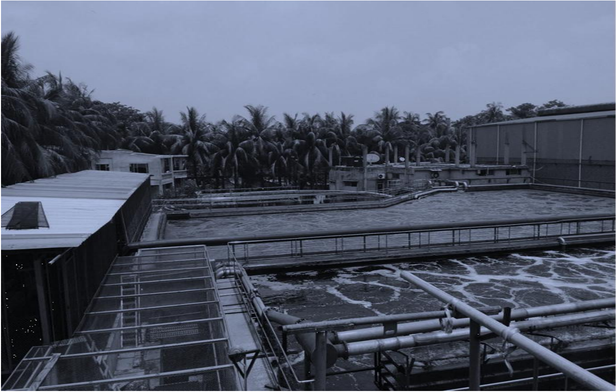
Effluent Treatment Plant
