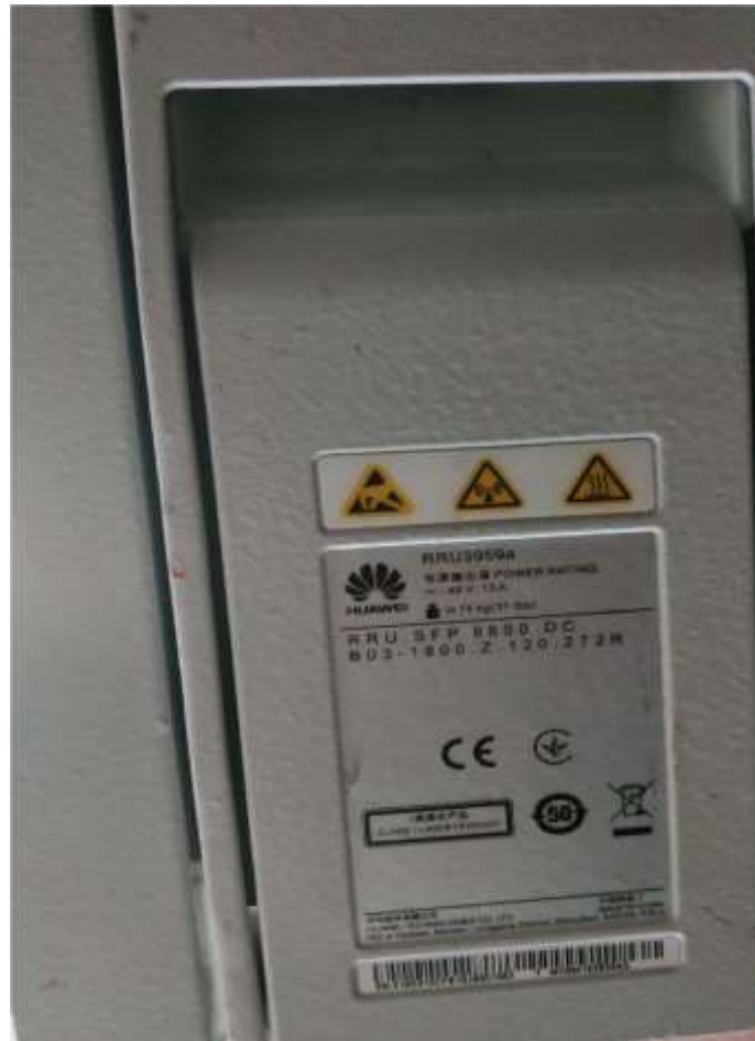
Fig-5.7: Remote Radio Unit (RRU)
