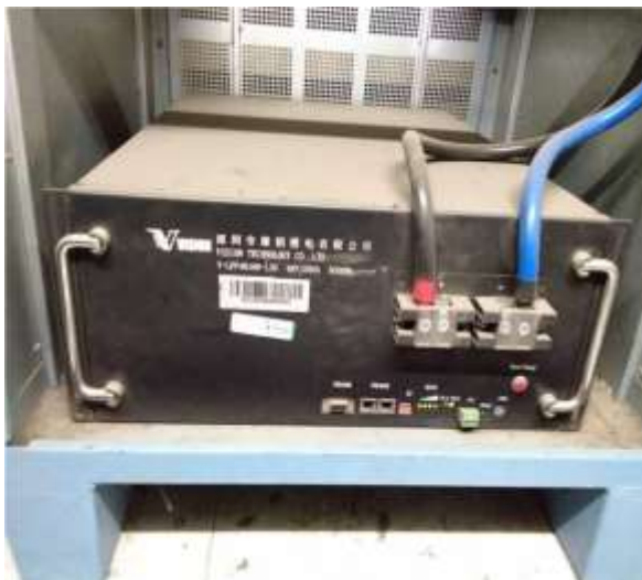
Fig-8.7: Battery & RRU Boards
