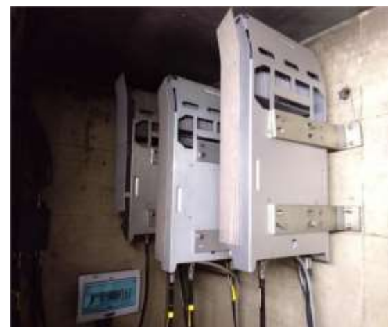
Fig-8.7: Battery & RRU Boards
