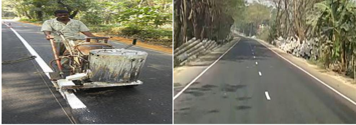
Figure:- 4.4 Road Marking
