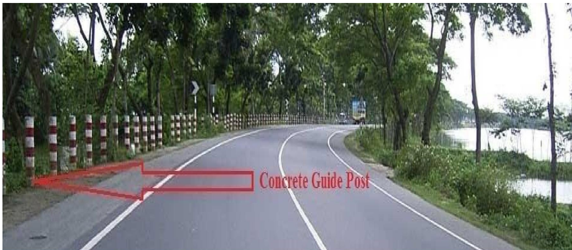
Figure: - 4.5 Concrete Guide Post
