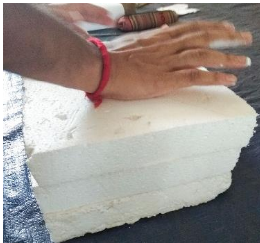
Figure: 5.1.9.2 Gluing Styrofoam's
