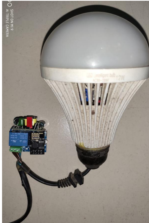
Figure 5.2: Installing Smart Home Electric circuit
