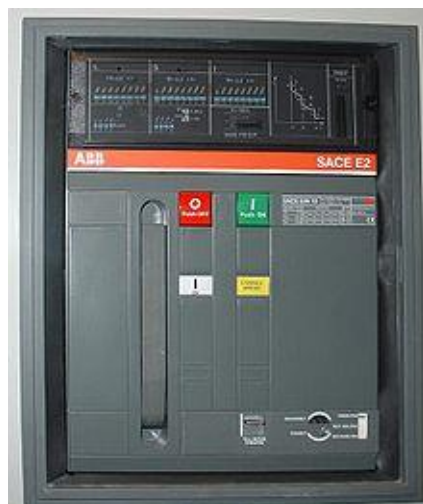
Fig7.3: Front board of a 1250 An air electrical switch made by ABB.
