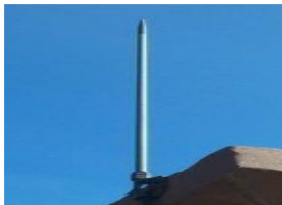
Fig6.1: An example of a standard, pointed-tip air terminal
