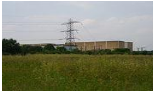
Fig2.3: Tottenham Substation set in wild parkland in North London
