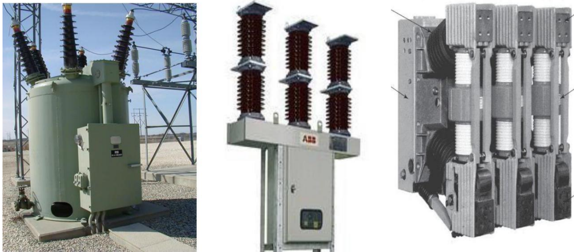
Fig 10.6: Oil, SF6 and Vacuum Circuit Breaker.
