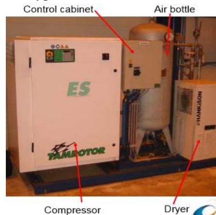
Fig: Control air system
