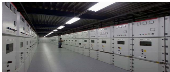
Fig: Generator Protection relay
