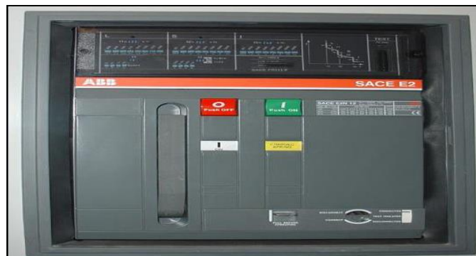
Fig 7.6: Air Circuit Breaker (ACB)
