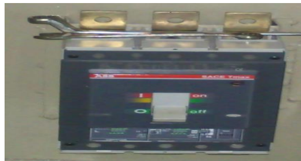
Fig 7.8: Molded Case Circuit Breaker (MCCB)
