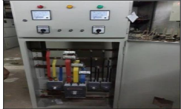
Figure 7.2: LT Switchgear
