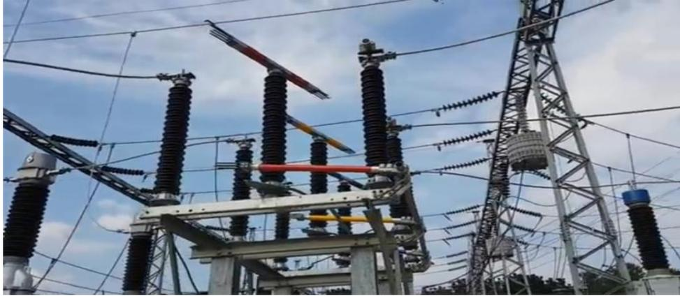
**Figure 3.15: Capacitor Voltage Transformer in Substation**
