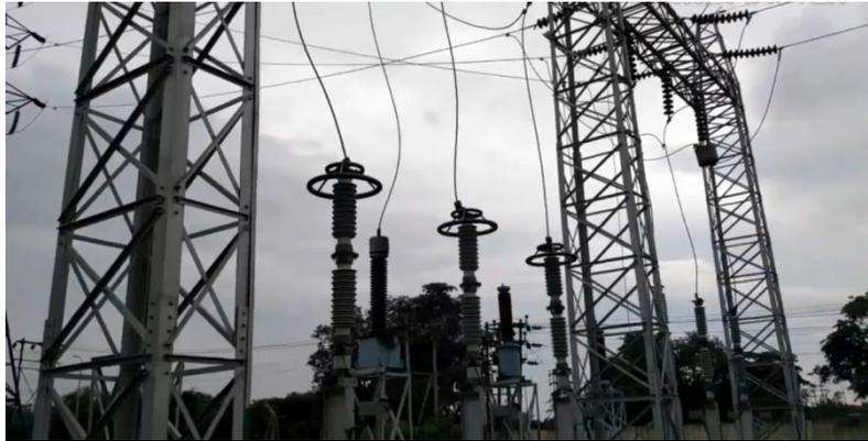
**Figure 3.13: Lightning Arrester in Sub-Station**
