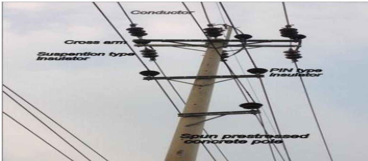
Figure 5.2: Fitting Of Distribution System
