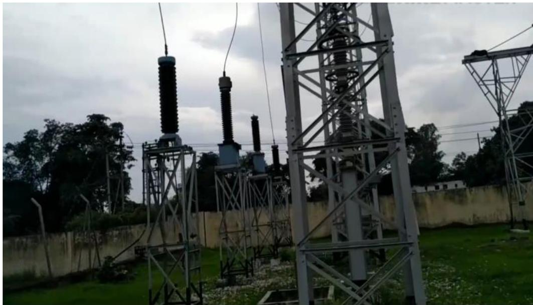
**Figure 3.3: Voltage Transformer**
