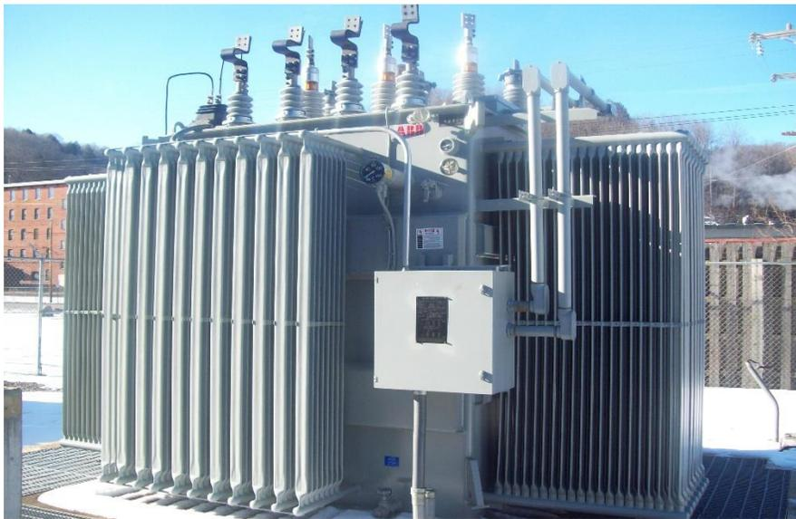
Figure3.8: Power Transformer in Sub-Station
