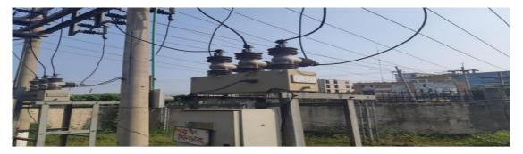
Figure 5.10: Feeding system of transformer in sub-station
