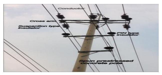
**Figure 5.2: Fitting Of Distribution System**
