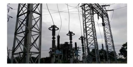
Figure 3.13: Lightening Arrester in Sub-Station
