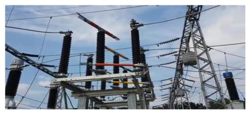
Figure 3.15: Capacitor Voltage Transformer in Substation
