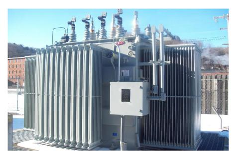
Figure 3.8: Power Transformer in Sub-Station
