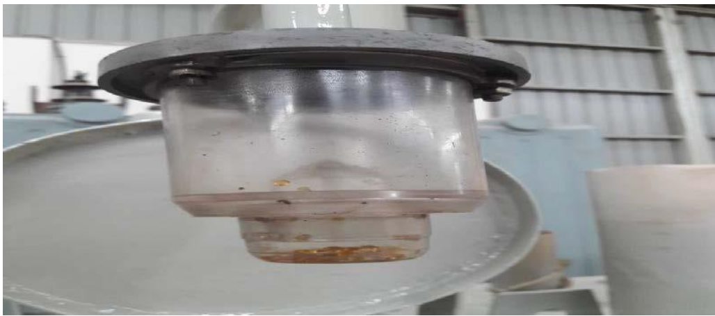
Figure 4.20: Construction of Silica Gel Breather
