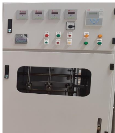
Figure 5.4: LT Switchgear [6]
