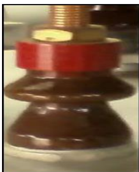
Figure 4.6: Pin Type Bushing
