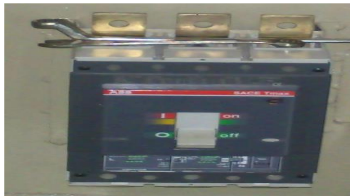
Figure 5.8: Molded Case Circuit Breaker (MCCB)
