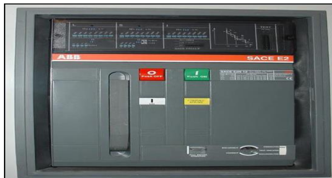
Figure 5.6: Air Circuit Breaker (ACB)
