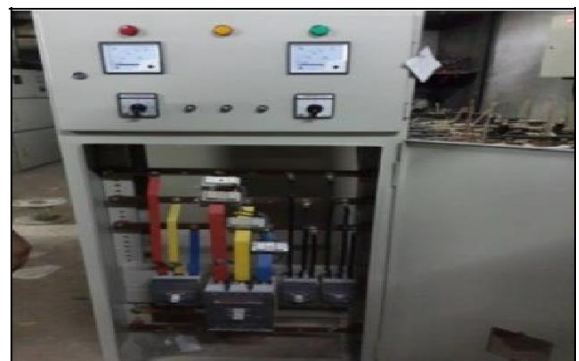
Figure 5.2: LT Switchgear
