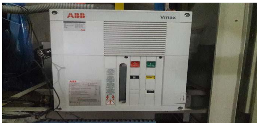
Figure 5.5: Vacuum Circuit Breaker (VCB)
