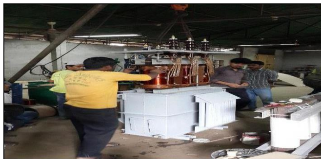
Figure 4.17: Placing Transformer inside the Tank
