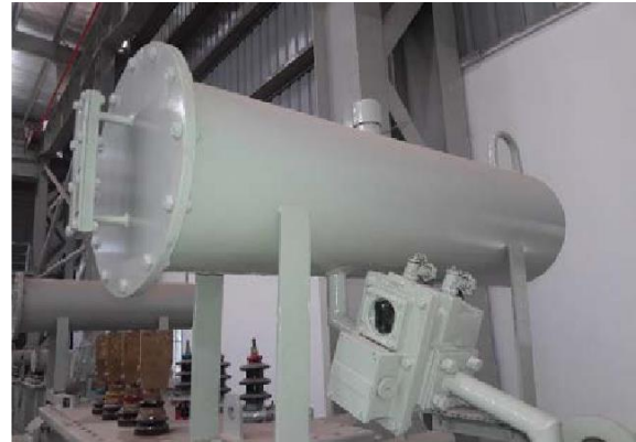
Figure 4.16: Conservator Tank
