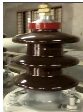
Figure 4.7: Shackle Type Bushing
