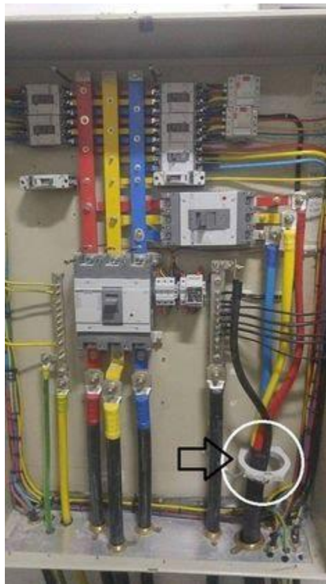
Figure: 2.5-DB board connection
