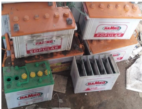
Figure 3.16: Wasted batteries due to lack of maintenance
