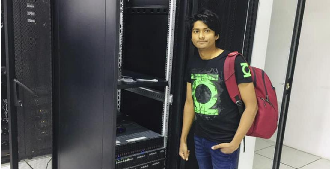
Figure 5.2.2: Datacenter Server Setup of FellowIO
