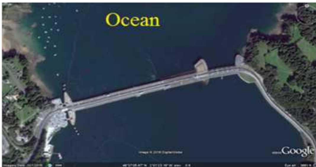
Fig 2.3: Top view of La Rance tidal power plant barrage (750m in length)
