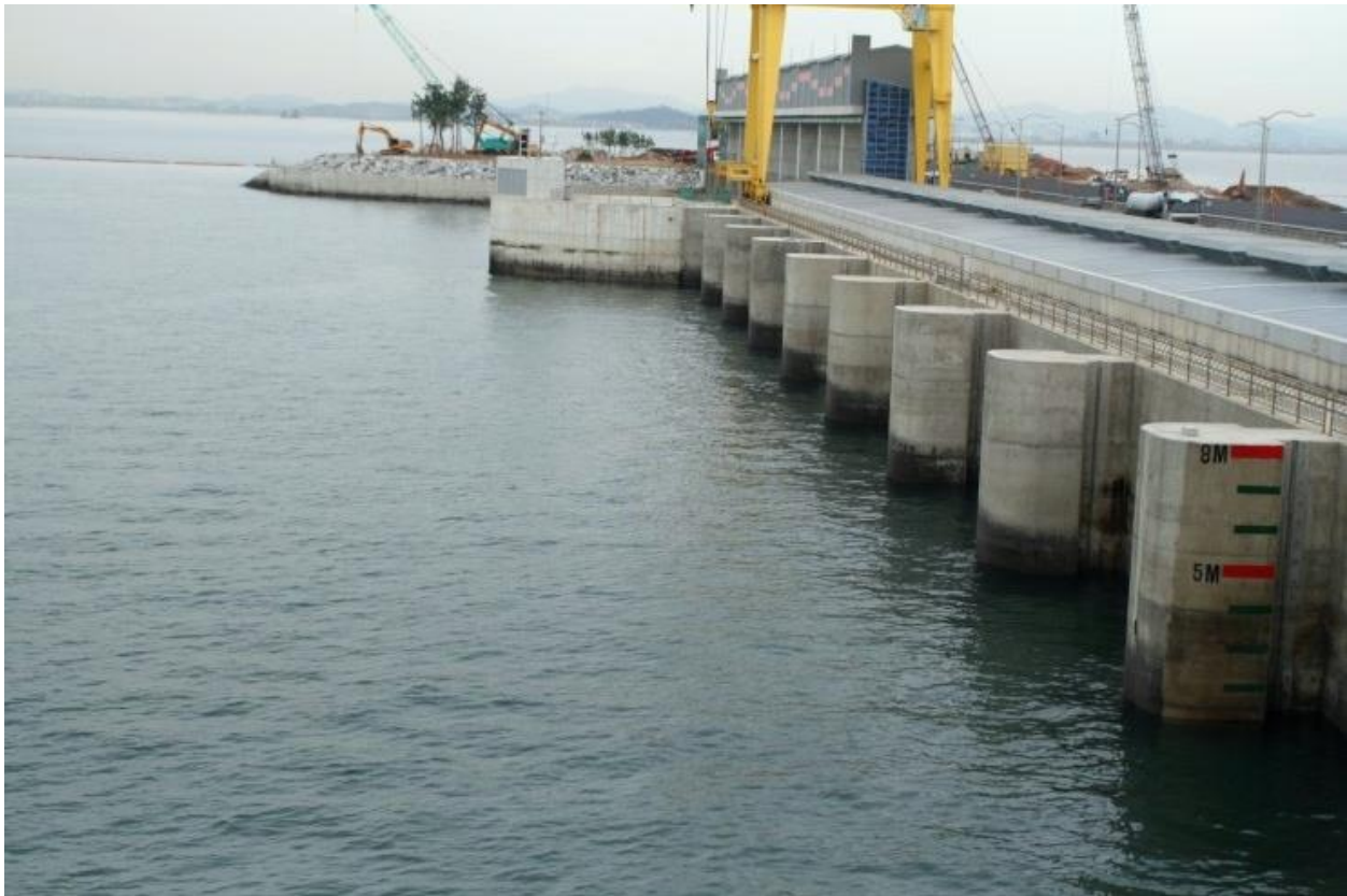
Fig 2.4: Shiwa Lake Tidal Power Station
