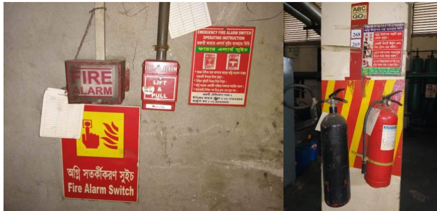
Figure 6.1: CO 2 fire safety cylinders for internal instrument protection in Liz Fashion Industry
