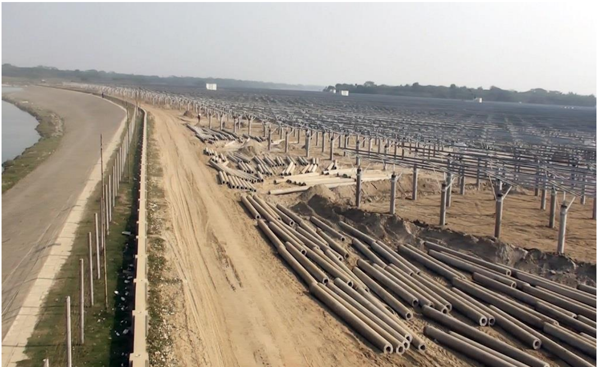
Figure 4.5.7: The solar-based power plant under construction in Mymensingh
