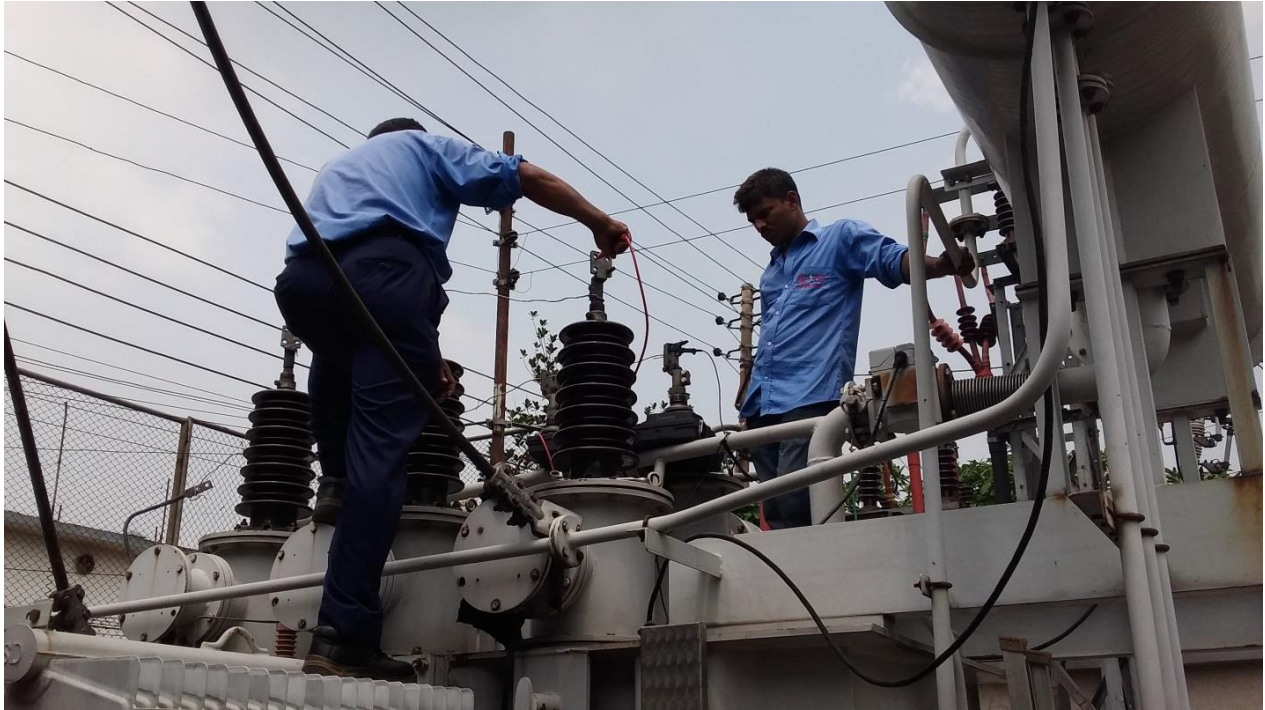
Figure 5.2: Maintenance of Digun 33/11 KV substation.
