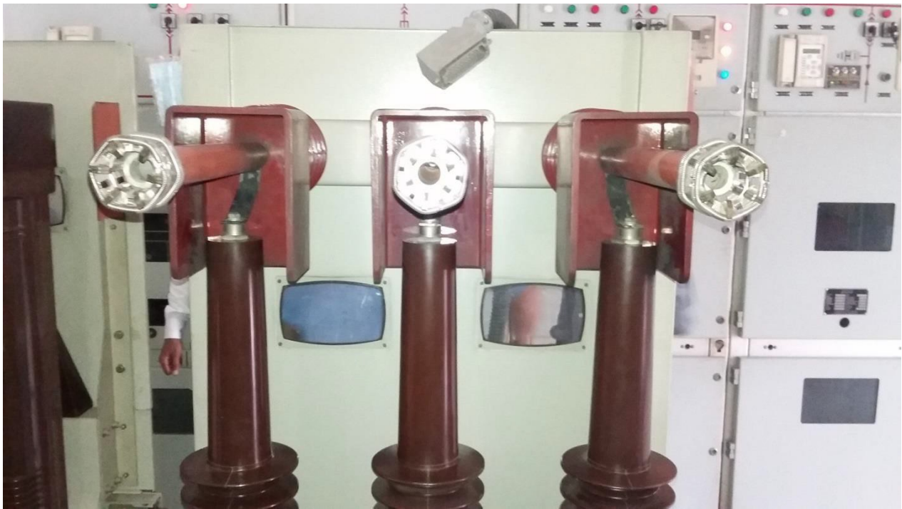
Figure 5.3: Checking insulation resistance between each winding & ground by using megar meter.
