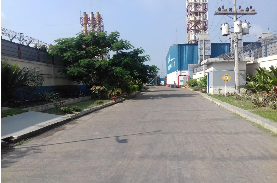
Figure 1.3: Overview of Narayanganj power plant
