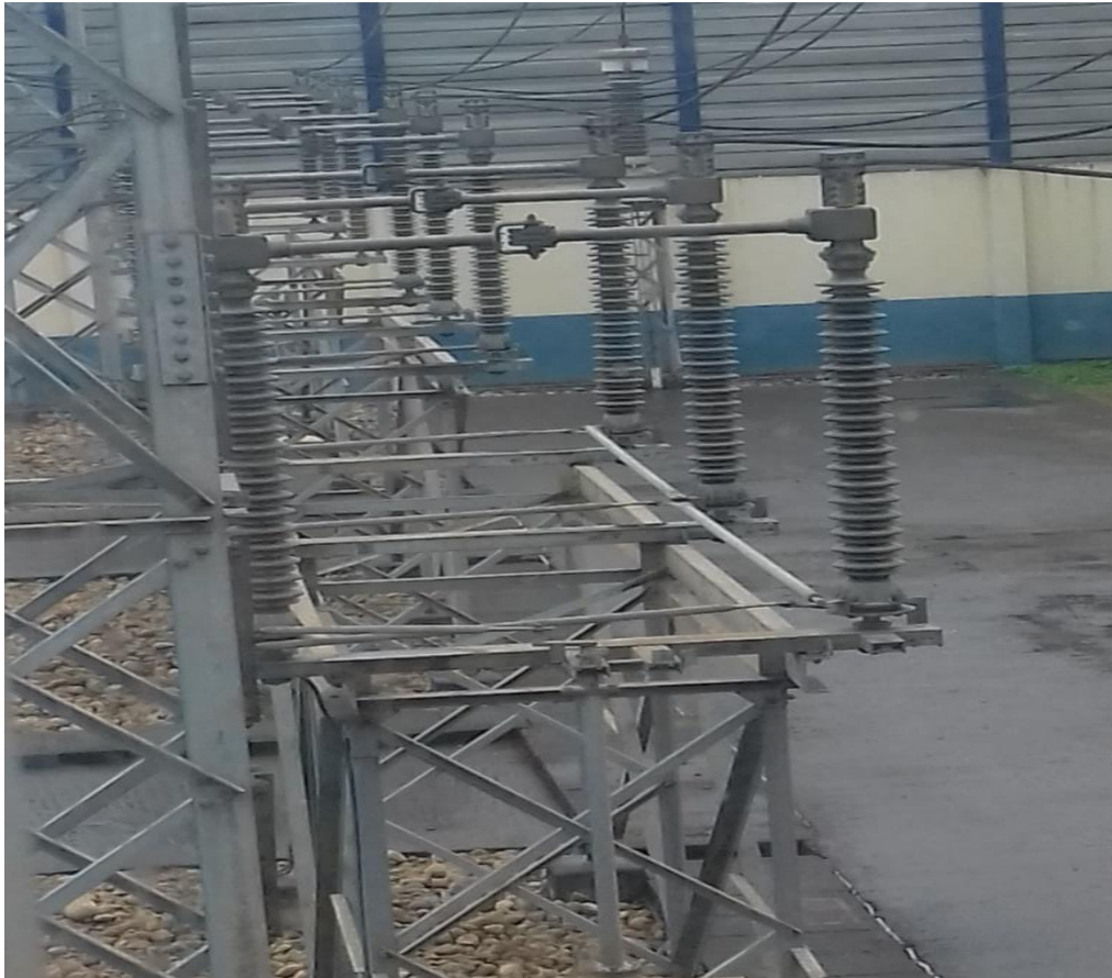
Figure 4.12: Disconnecting Switch
