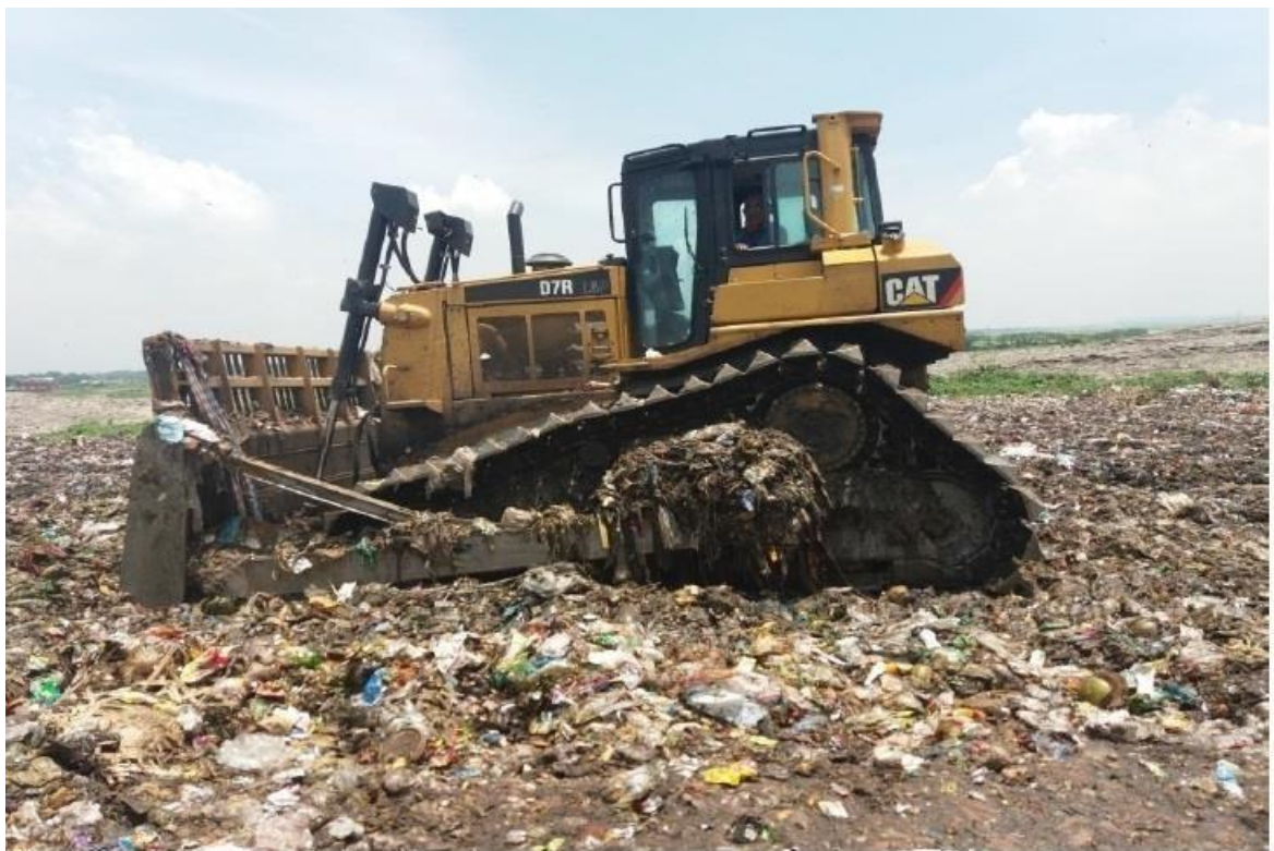
Figure 3. Compaction of waste by chain dozer at Amin Bazar landfill
