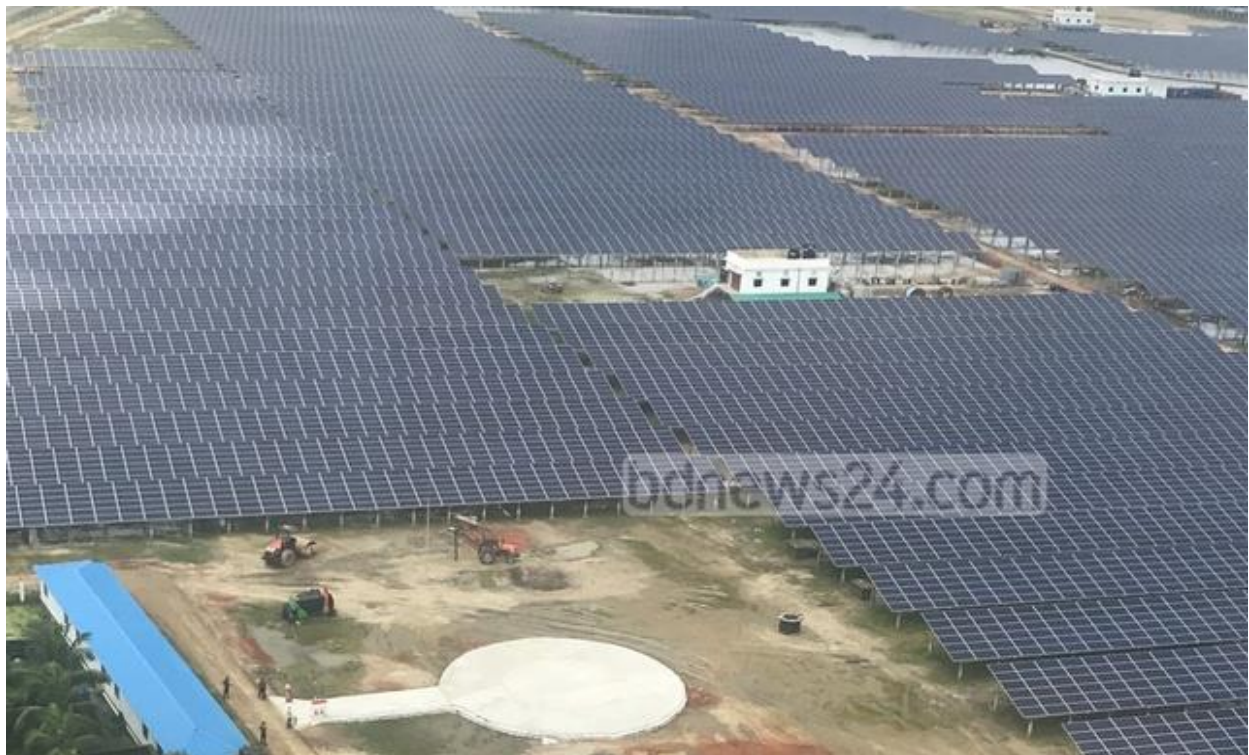
Figure: 2.1: Bangladesh's largest solar power plant in teknafs.
