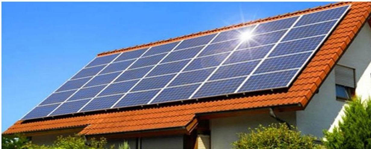
Figure 1.1: Solar rooftop system
