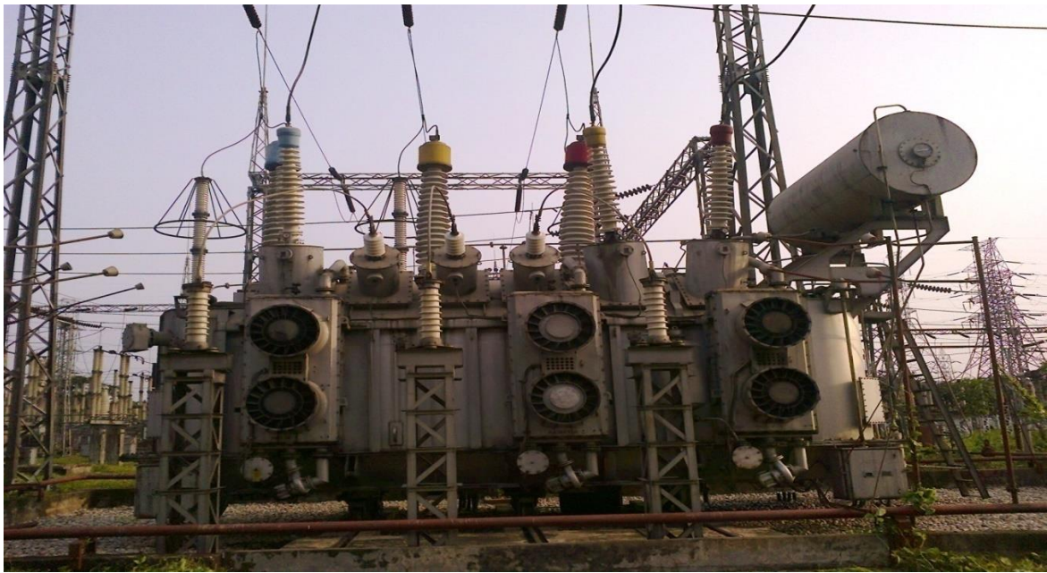
Fig 8.1: Unit Transformer
