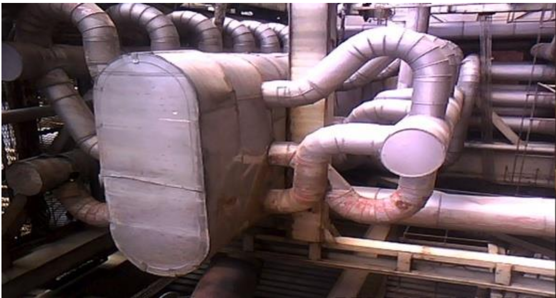
Fig 5.11: Condensing Plant.
