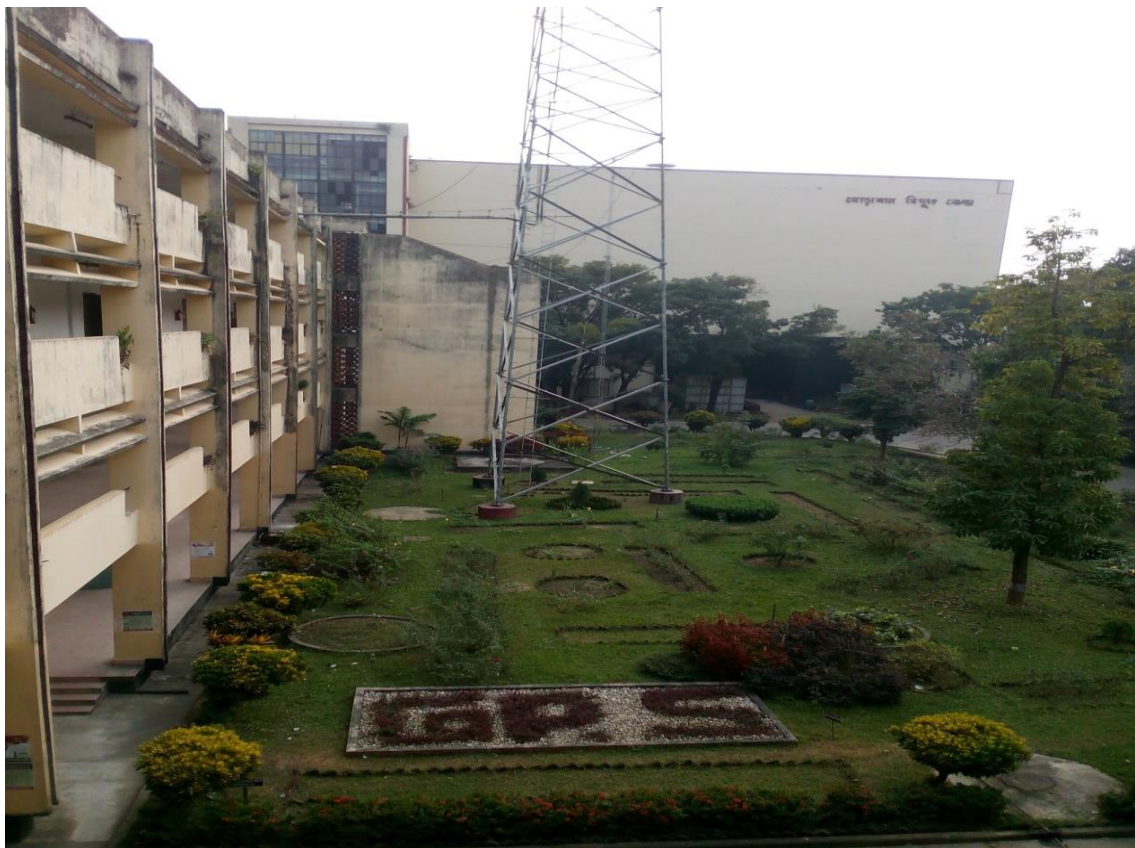
Fig 2.1: Ghorashal Power Station
