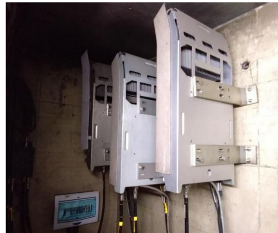
Fig-6.5: Battery & RRU Boards
