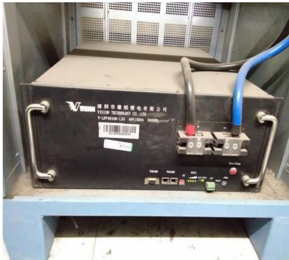
Fig-6.5: Battery & RRU Boards
