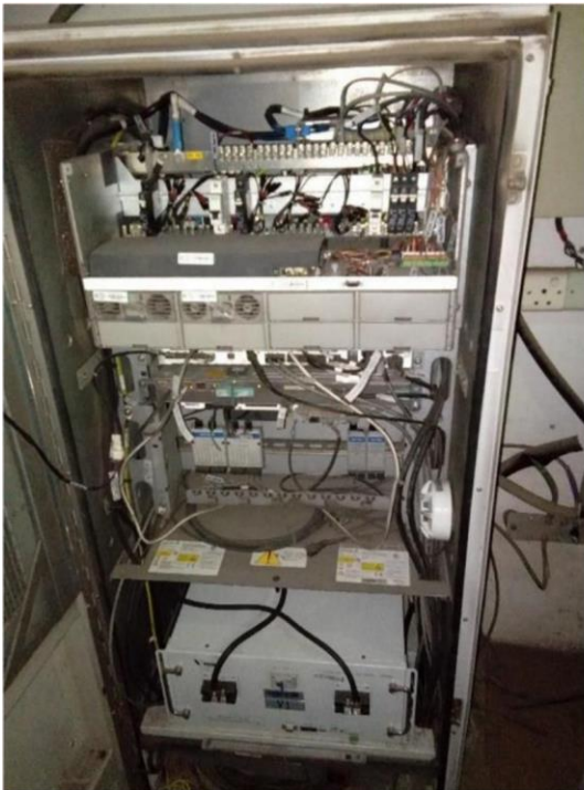
Fig-6.3 - RX Rack with switches & Battery And RRU Connector Board(BTS)
