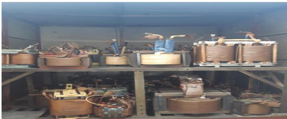
Figure 4.9: Heating Chamber of Transformer
