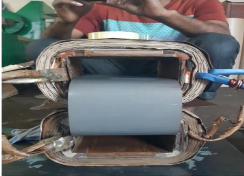
Figure 4.8: Transformer repairing in workshop
