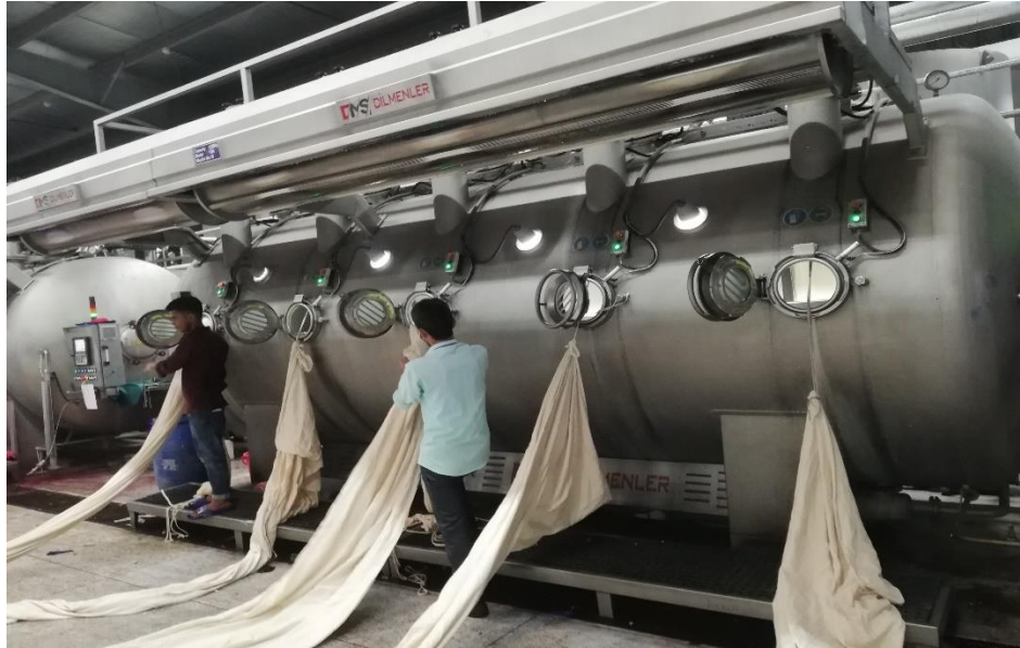
Figure no. 2.3: DILMENLER dyeing machine for pre-treatment.
