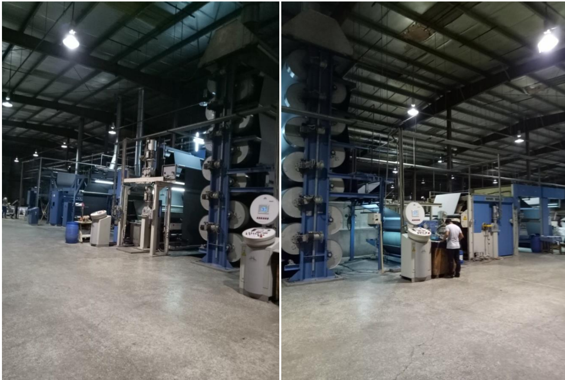
Figure17: over view of finishing machine
