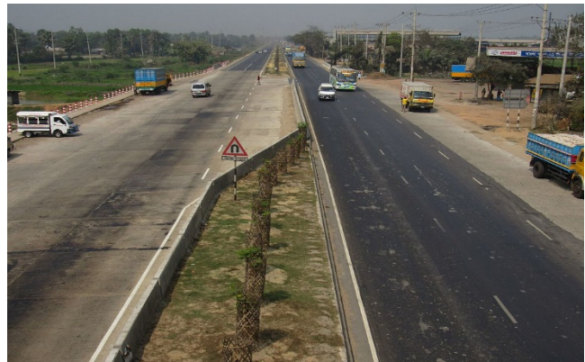
Figure 3.2: Dhaka-Chittagong Highway after expansion
