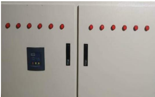
Fig: Power Factor improvement Plant (PFI).
