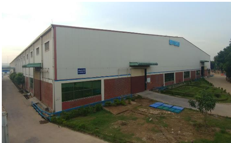
Fig 1.2: Factory Shed: Refrigerator Unit
