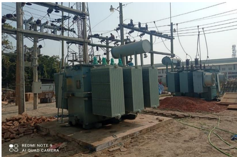
Fig 5.2: 10 MVA Transformer
