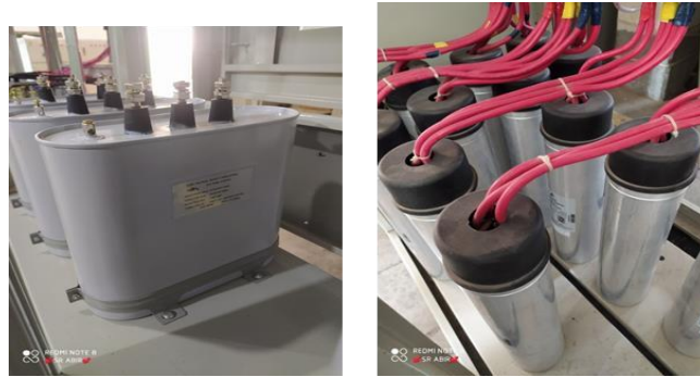
Fig: 9(b): Capacitors
