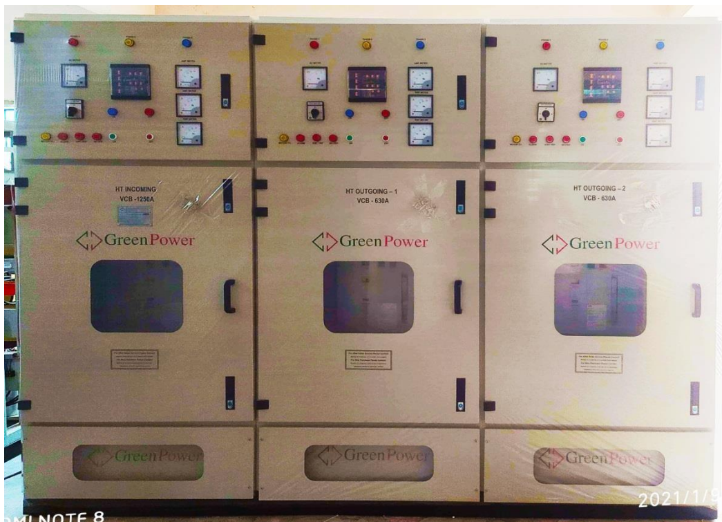
Figure 5.1: Ring Main Unit (RMU)
