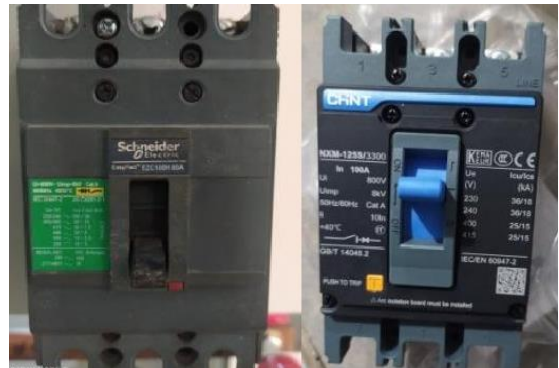
Figure: 4(a) MCCB (Schneider & ChiNT)
