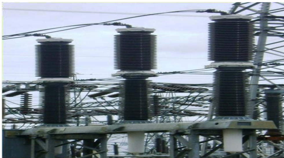
Fig. 6.3. Bus coupler at GPS
