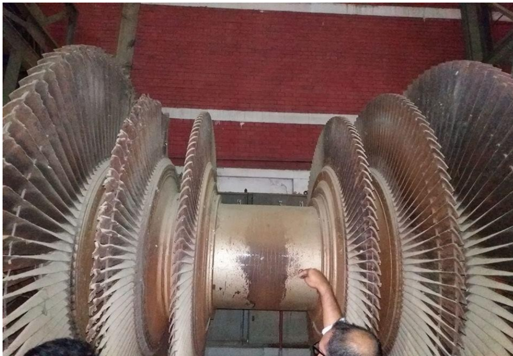
Fig. 4.4. Rotor of low pressure cylinder at GPS
