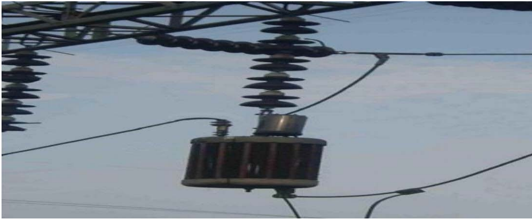
Fig. 6.8. Wave trap at GPS
