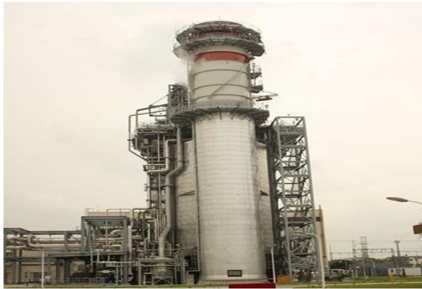
Fig. 2.6. Chimney at GPS unit-4
